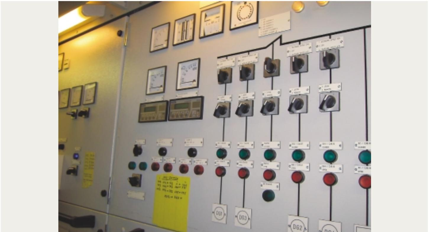
Fig. 6 – Back-up control at the main switchboard in case of PMS failure.
