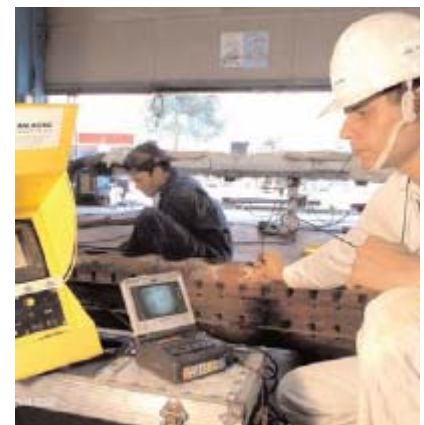
Examination of boiler by means of fibroscope to check for cracks.
